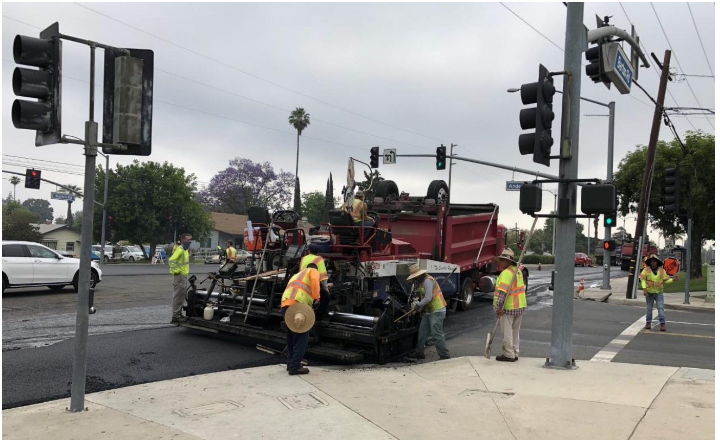
Pavement Rehabilitation at Barton Road
