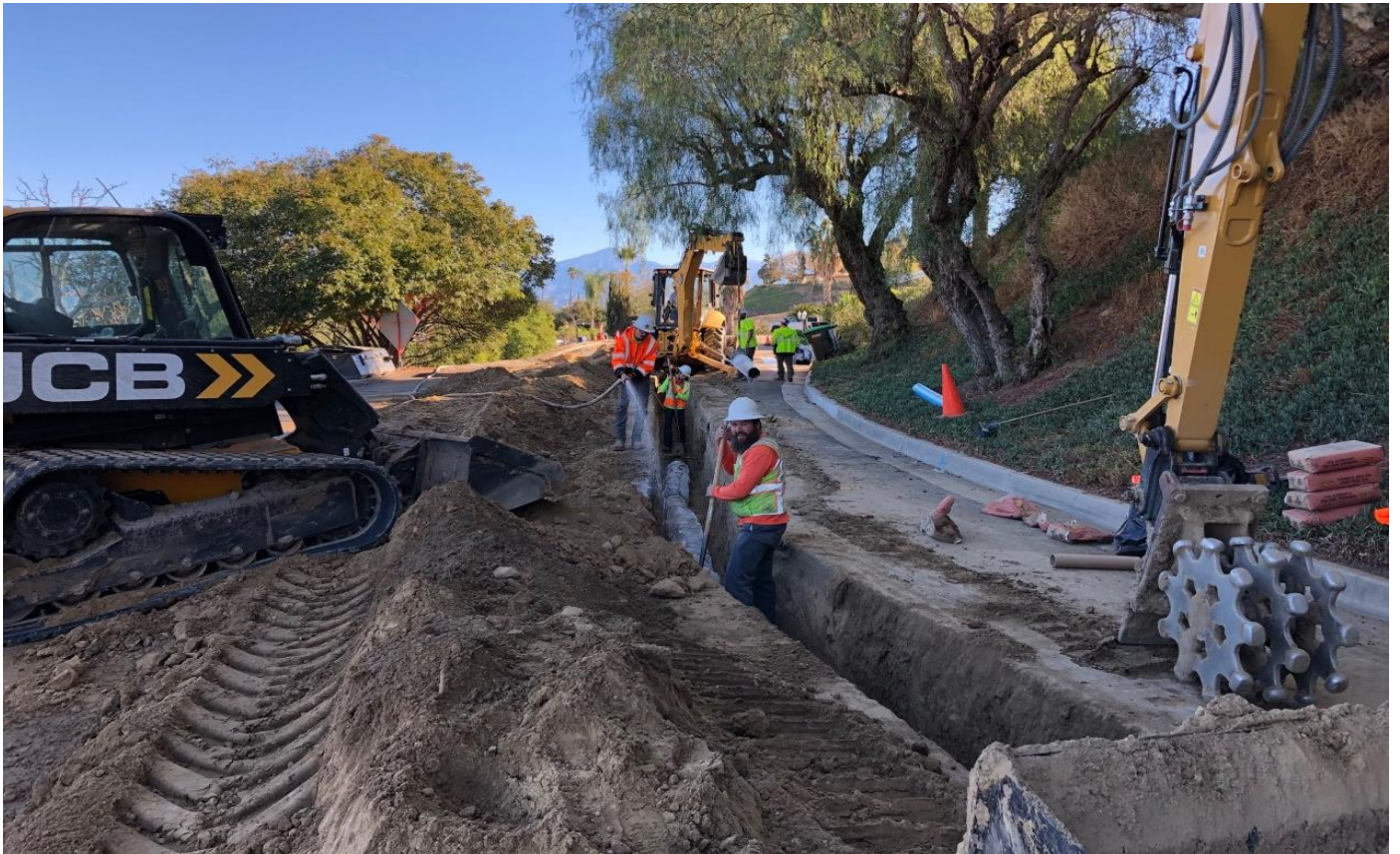
The installation of waterline at Lawton Avenue
